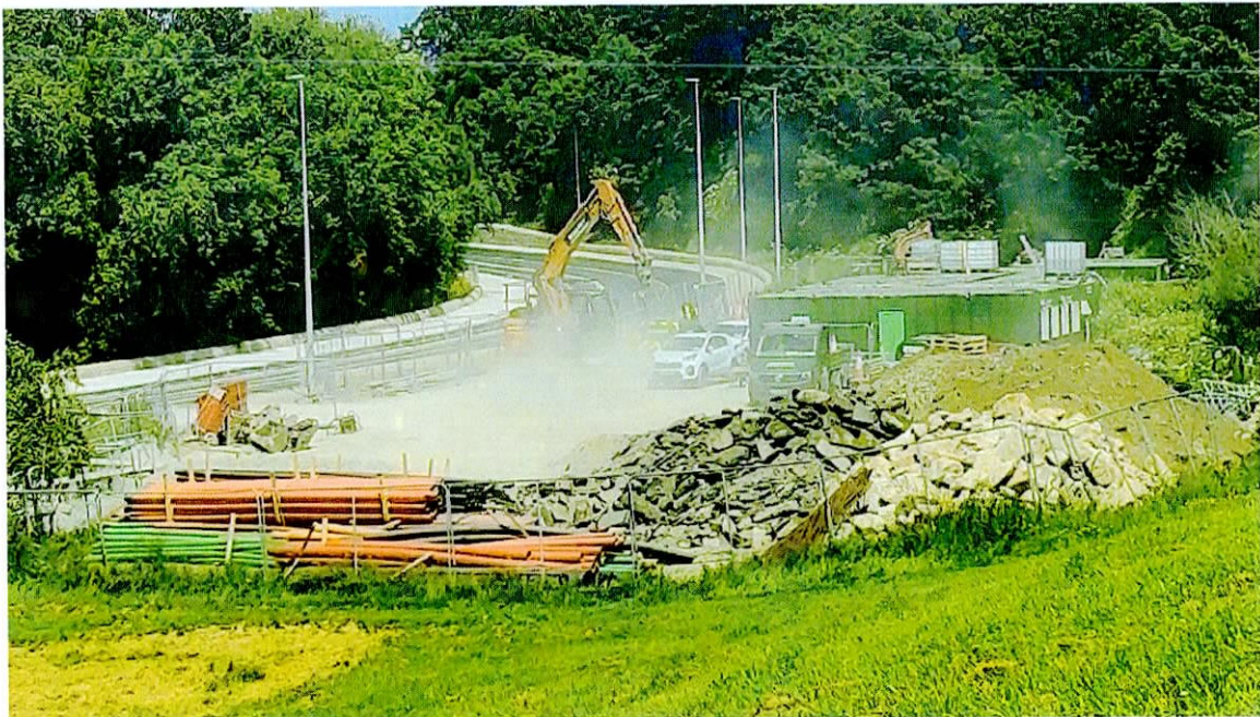
Fig 1.5 30/05/2023 - Dust from the existing construction site for the Greenway
